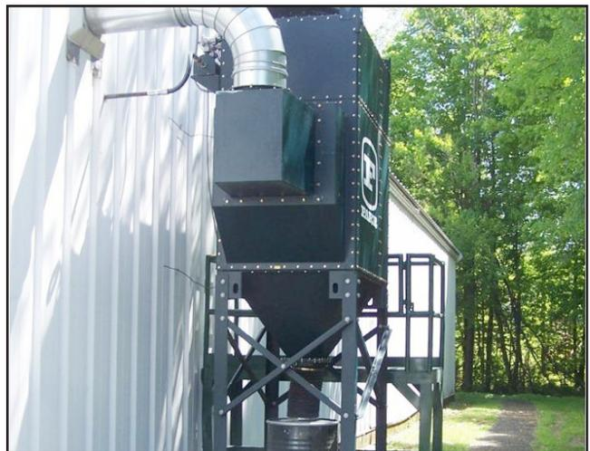
GS6 located on the outside connected to the saws inside the building.
