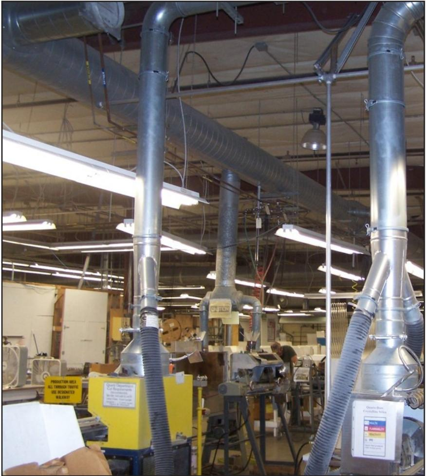
Ducting from the saws inside the building to the Farr dust collector outdoors.
